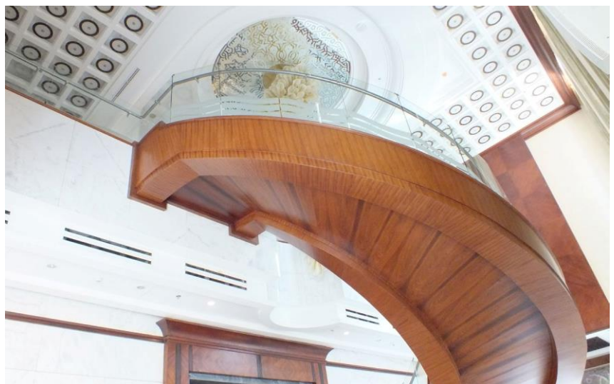
Wooden Cladding & Stainless Steel With Glass Handrails
