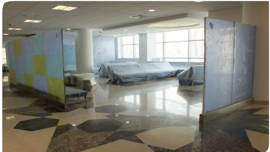
Hospital of the King Saud University (3 form Partitions Decoration)
