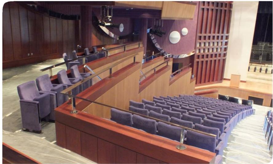
Wooden Cladding & Stainless Steel Handrails
