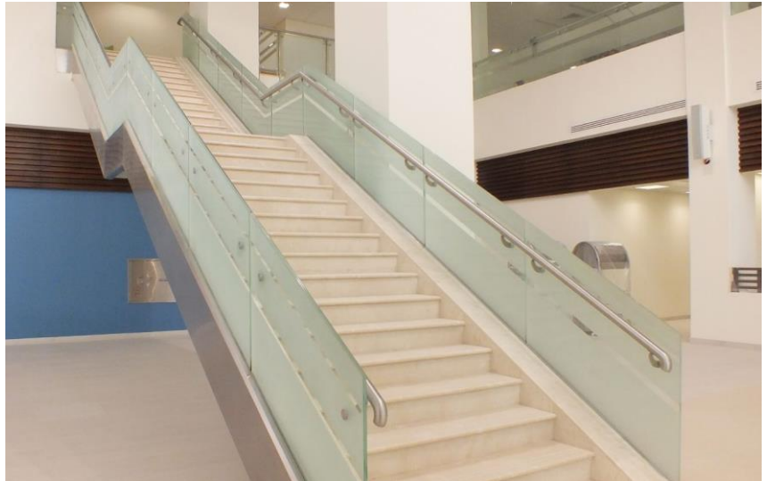
Laminated Glass With Stainless Steel Handrails
