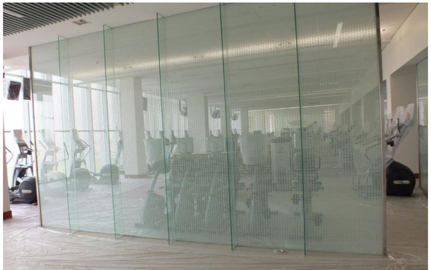
Laminated Printed Glass Partition
