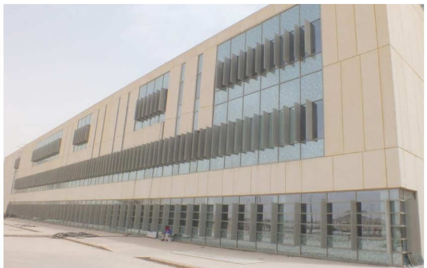
Research center (Curtain wall)
