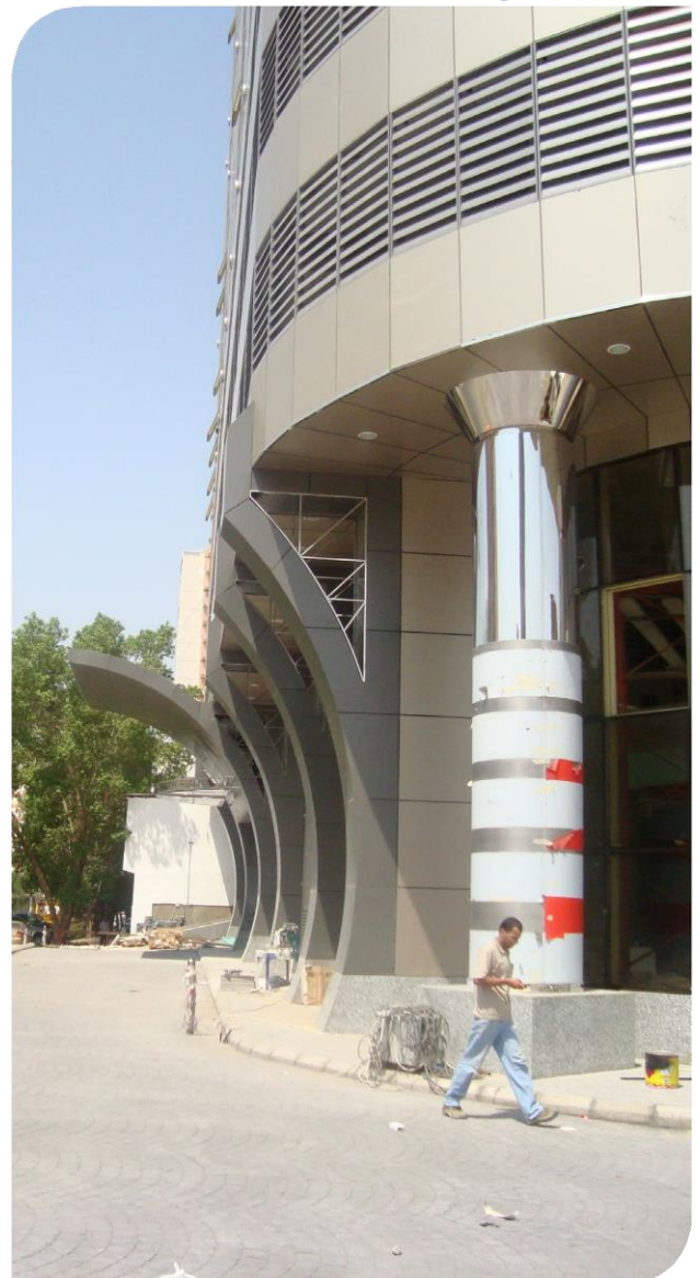
Stainless Steel Columns Aluminum Cladding
